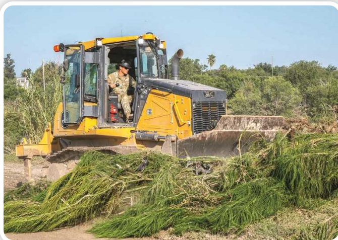
TEXAS ARMY NATIONAL GUARD AND TEXAS STATE GUARD SERVICE MEMBERS supporting #OperationLoneStar cleared debris caused by recent flooding before replacing barriers along the Rio Grande River.
